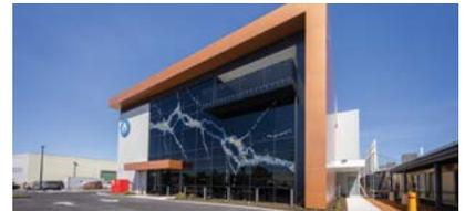
The eastern-facing glass wall is made of low emissivity (low-e) glass.
