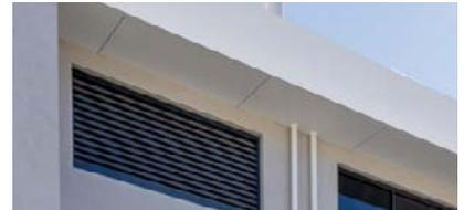
Cost-efficient, lightly coloured concrete slabs were used for heat reduction on building envelope. Portrait orientation of the window allows access to the lab level for larger machines and maintenance.
